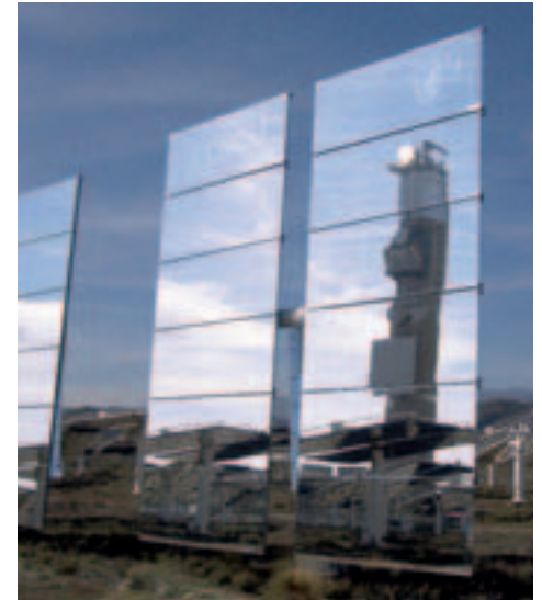
PSA-CESA | Solar thermal central receiver
